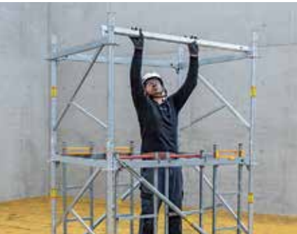
The ledgers can be quickly mounted from a safe position. The self-securing ledger assembly with the Gravity Lock increases the level of working safety.
